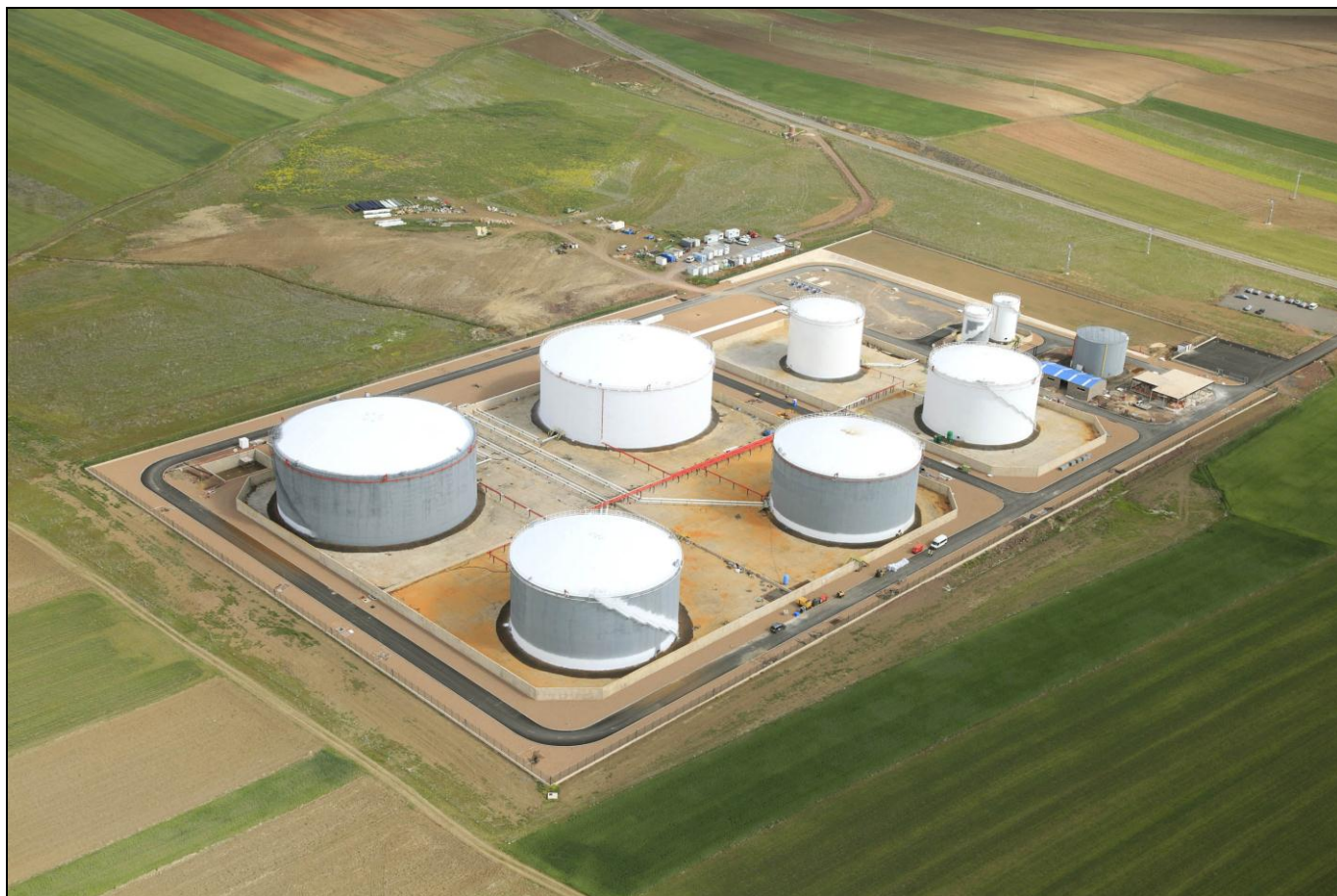
Tanques (2) almacenamiento Gas Oil ( \varnothing 56 \times 20 mtrs. Total 98.520 m 3 ) para C.L.H. (I.A. Almodovar del Campo)
